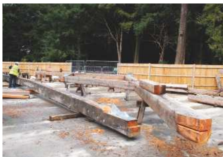
The horizontal timbers are made from Corsican pine and are hewn by hand to create a curve
